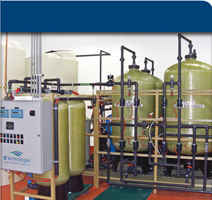
▲ 2-Bed High Capacity Water Recycle System
