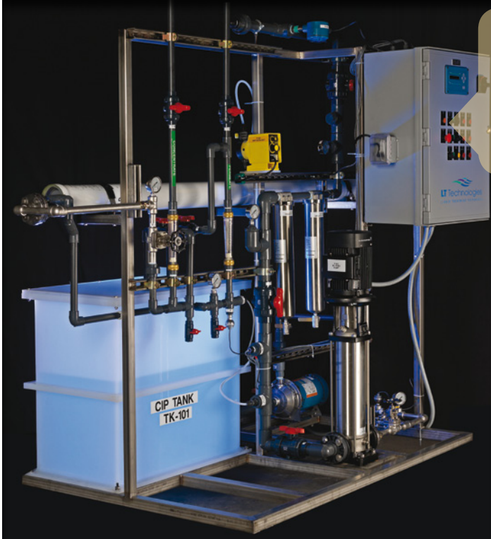
▲ Nanofiltration chemical recovery system
