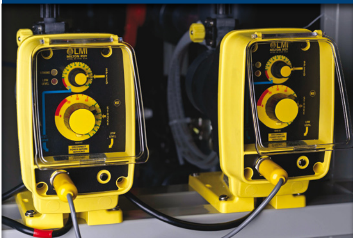
▼ Chemical Injection Pumps
